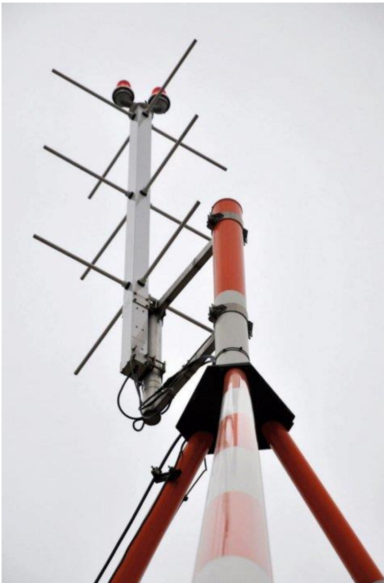
GBAS antenna at Frankfurt Airport. (DFS)
